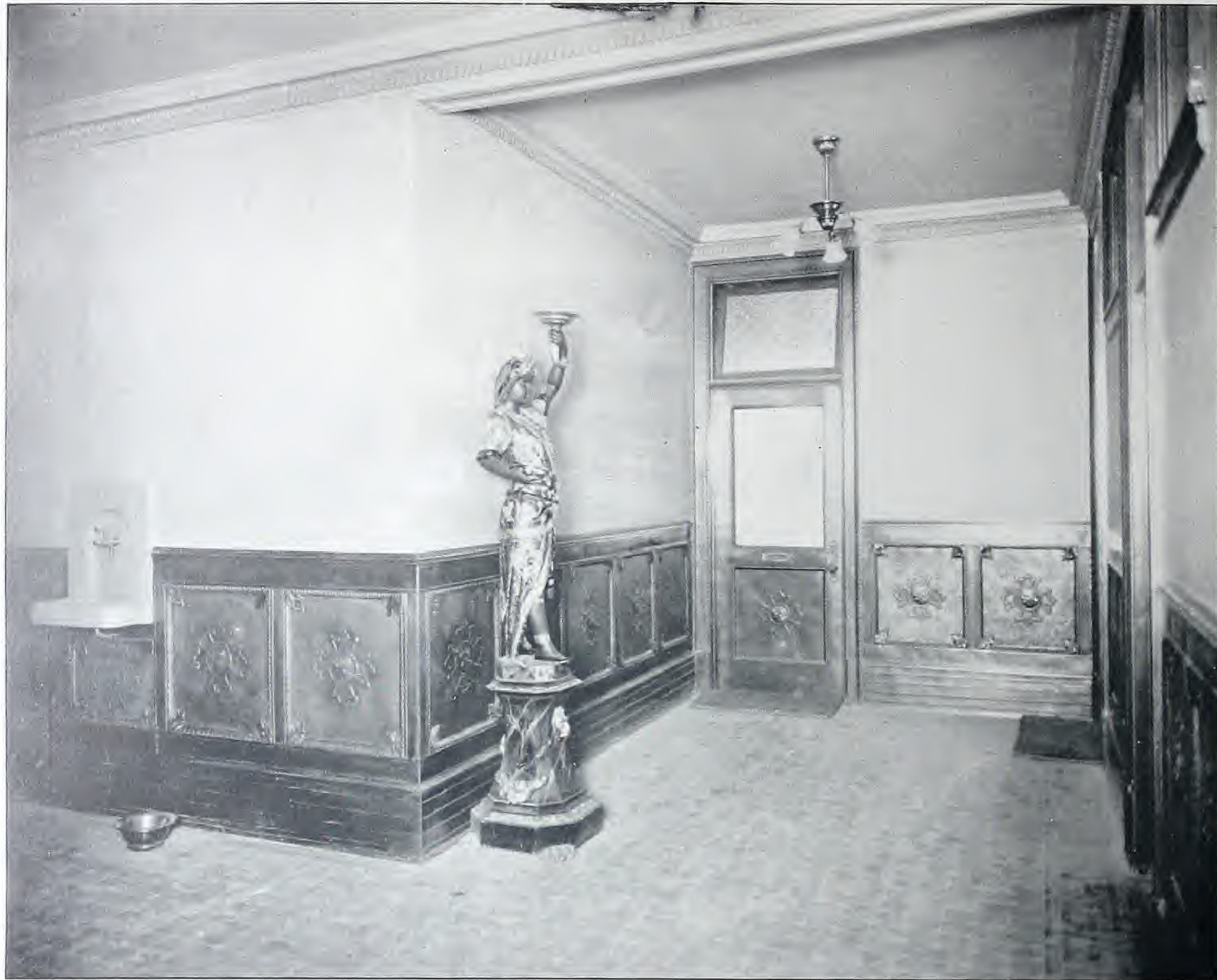
Fig. 145. —Interior View, Temple Building, Toronto.
